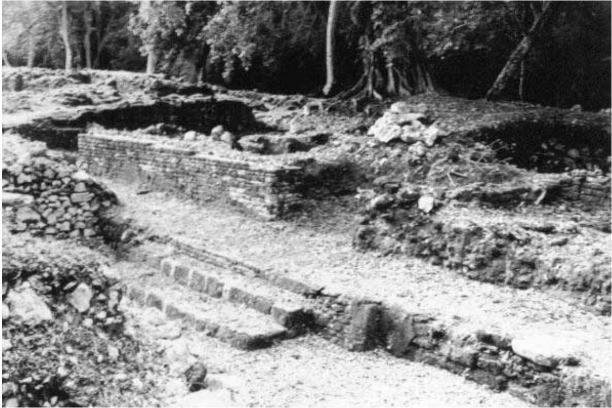
Figure 2:6. Photograph of Structure N10-28 taken before the 1999 excavations.
