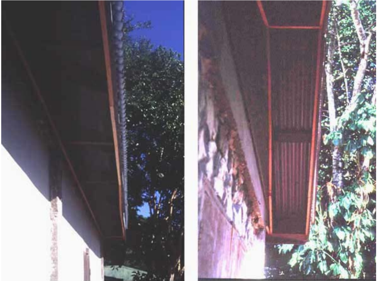
Figure A1:11. Bodega soffit after screening.
