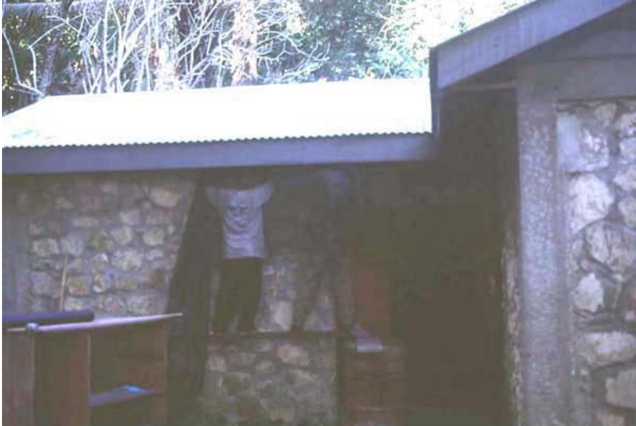
Figure A1:13. Federico and Israel installing screening beside bodega entrance.
