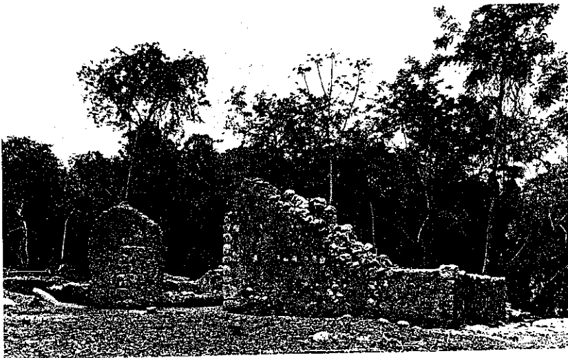
The remains of the church at Lamanai. Only the apse was made of masonry; the nave, which covered much of the left foreground, was constructed of perishable materials.
