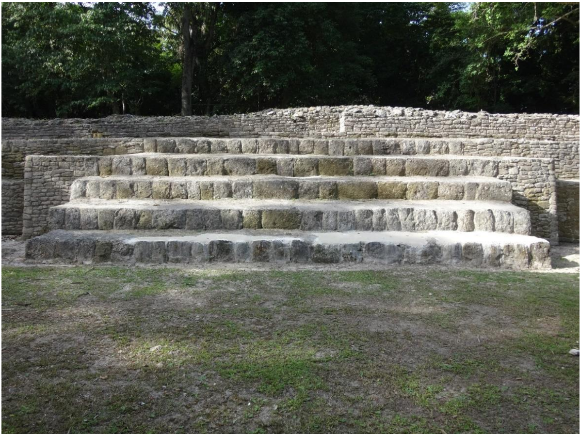
Figure 6.39. Structure N10-15 south stairs (photo by Karen Pierce, 2014).
