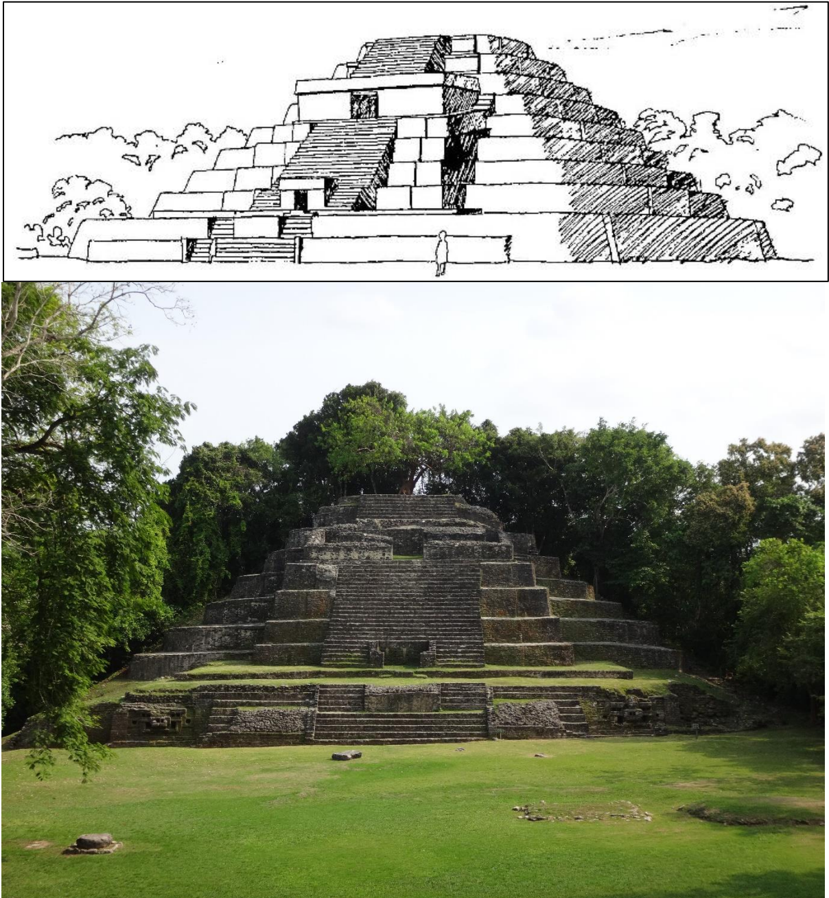
Figure 5.11. Above: Lamanai Structure N10-9 Late Classic (A.D. 7 th –8 th centuries) phase (Pendergast 1981a:35, figure 5). Below: Structure N10-9 after 2002 TDP reconstruction (photo by Karen Pierce, 2014).
