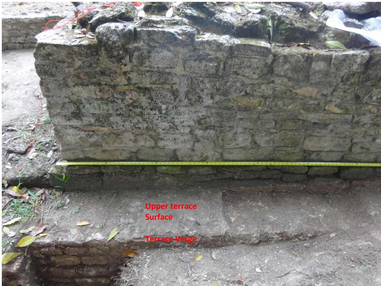
Photo 3808 (May 16) Looking south. The following is a series of photos (through 3815) going from east to west on the north side the N10-15 1 st north wall showing basal molding (tape measure rests on basal molding) and the upper terrace verge (edge).
