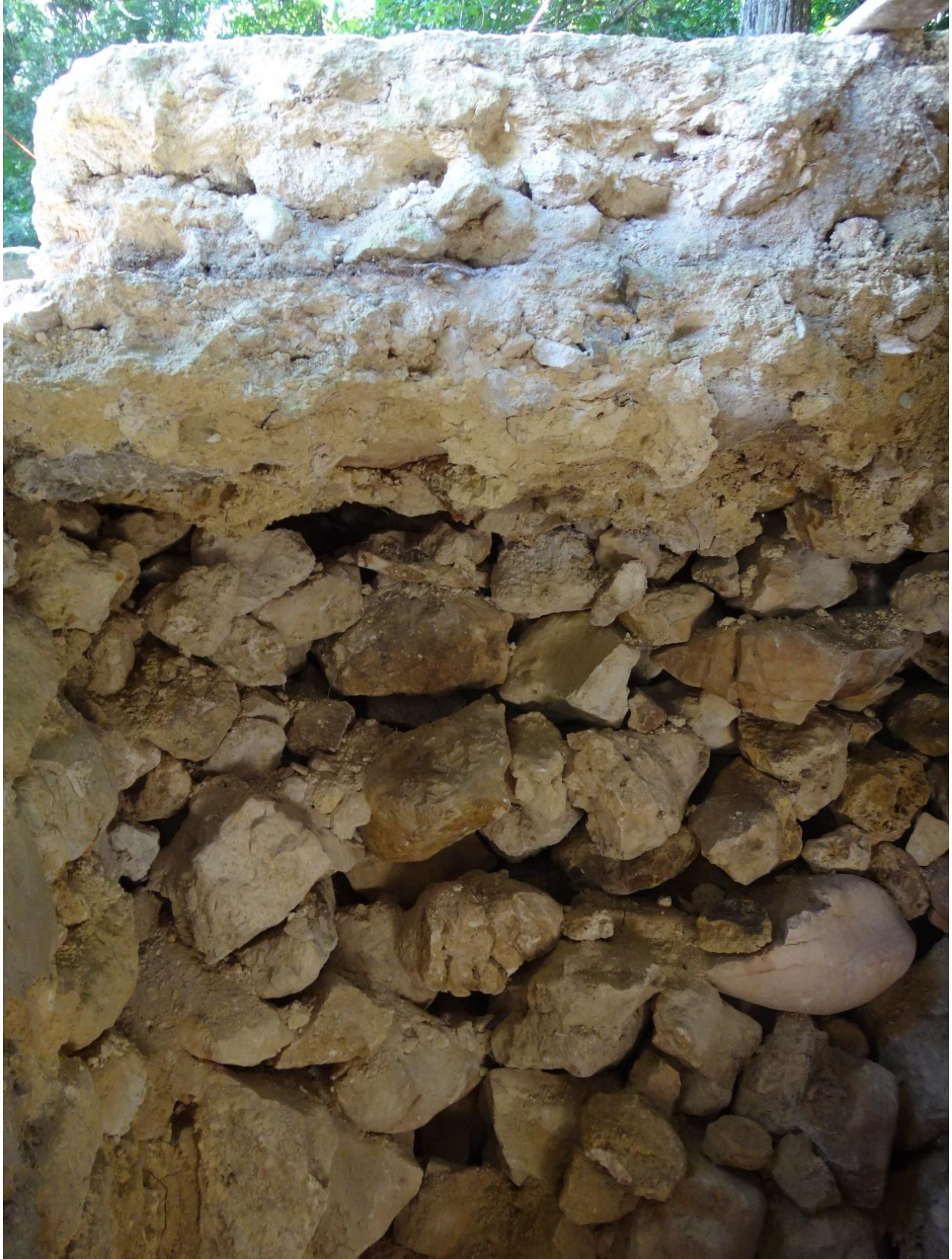
Photo 5683 (June 20) Looking west. Floor core over dry-laid boulder core (see previous phot for orientation).
