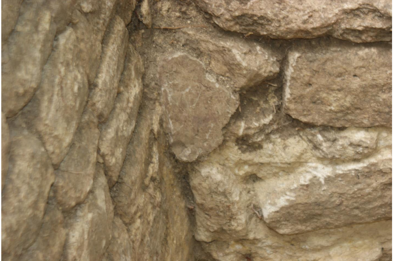
Photo 1934 (May 21) Looking West. Note patch of reddish (?) plaster on end of steps.
