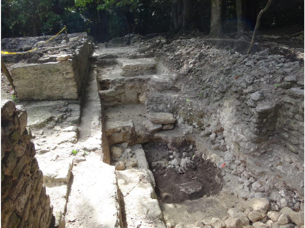
Photo 6234 (June 28) Looking west across N10-15 2 nd . The north wall and north door of N10-15 1 st is on the left. Backfilling and rebuilding the lower step.
