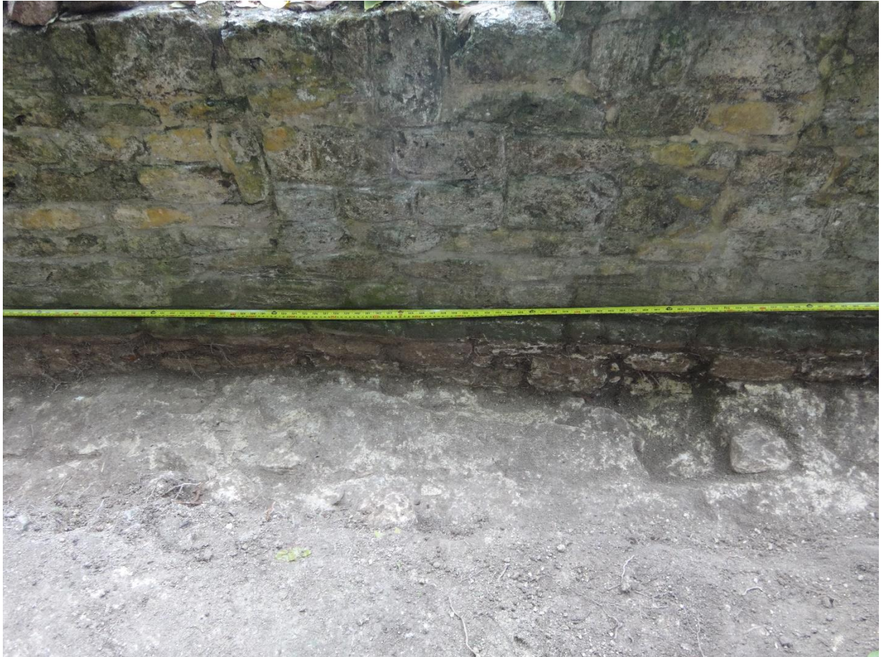
Photo 3812 (May 16) Looking south. Series of photos (through 3815) going from east to west on the north side the N10-15 1 st north wall showing basal molding and upper terrace edge.
