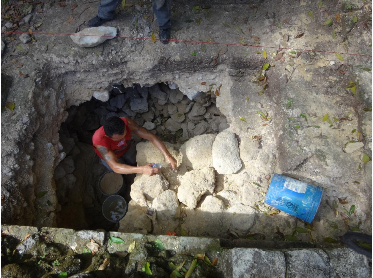
Photo 4450 (May 23) Looking north. Rebuilding buttress unit.
