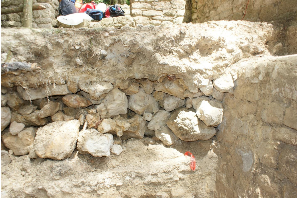
Photo 1971 (May 21) Looking East. Note patches of grey plaster on the terrace face.
