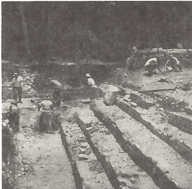
Fig. 1. Excavation in progress at the east end of "Ottawa"; the men are removing Boulders core from the face of Snow.
